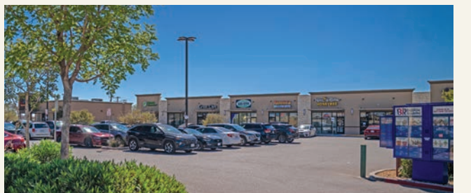
Emerald Park Plaza Located at the corner of Eastlake Boulevard and Emerald Park Drive
